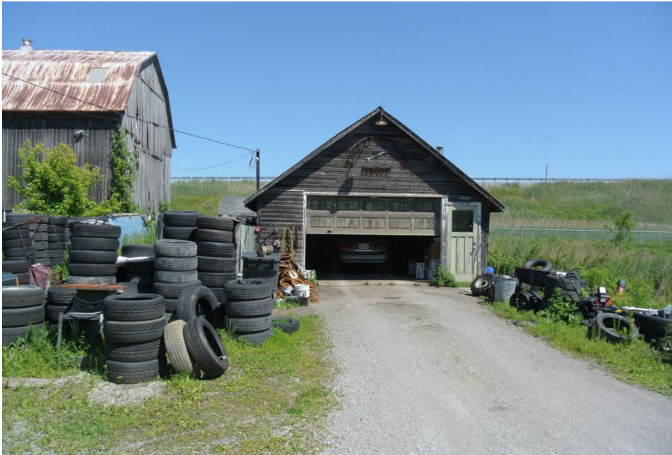
Plate 3: South elevation of garage at 8119 Reesor Road.
