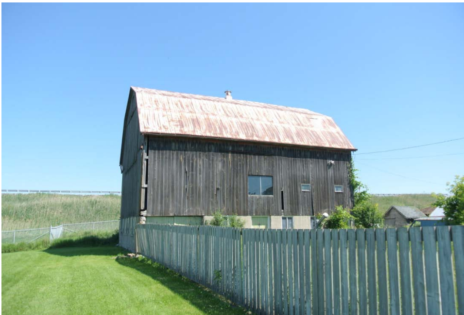
Plate 2: South elevation of barn at 8119 Reesor Road.
