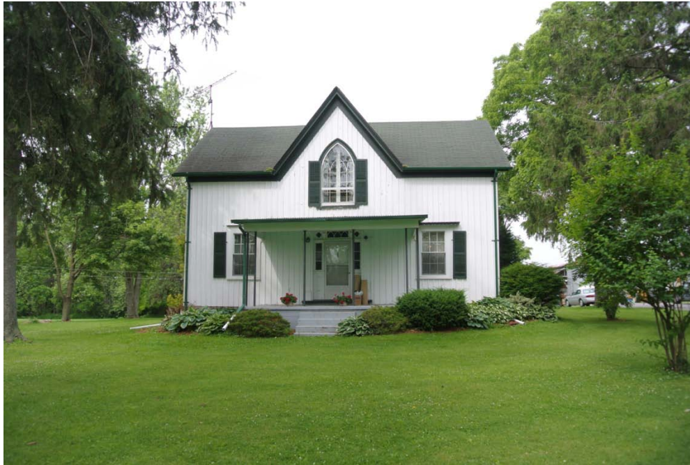
Plate 1: Front (east) elevation of 80429 Reesor Road.
