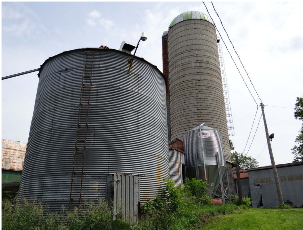
Plate 3: South elevation stave silo and representative modern corrugated metal silo, part of the granary complex at 8042 Reesor Road.
