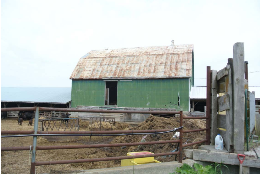
Plate 2: South elevation of barn at 8042 Reesor Road.
